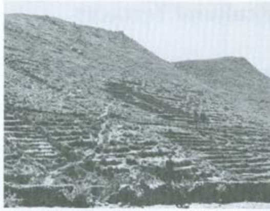
Fig. 2. Valley-side walled terraces. Cultivated terraces line the slope below a contour canal. Abandoned and semi-restored terraces are above.
