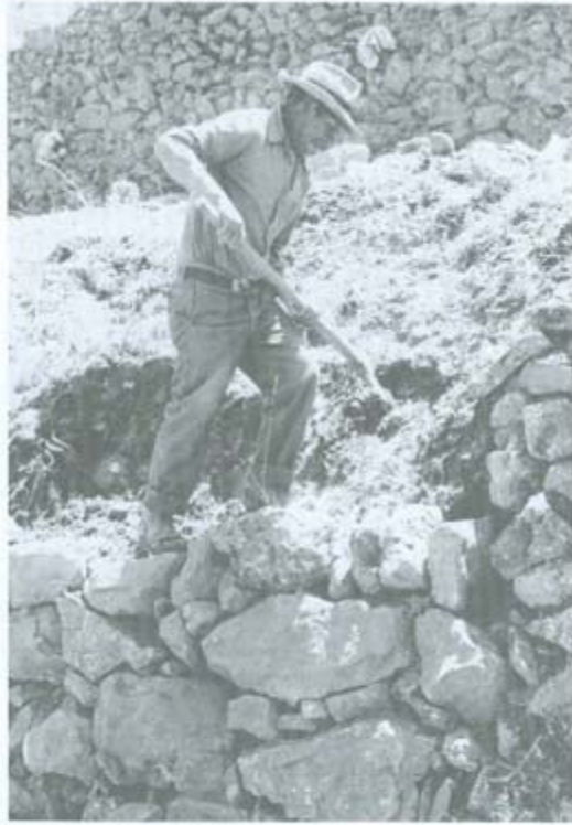
Fig. 5. Farmer standing upon half-completed wall, moving earth downward to fill in behind the stones. Note the jig-saw masonry style.
