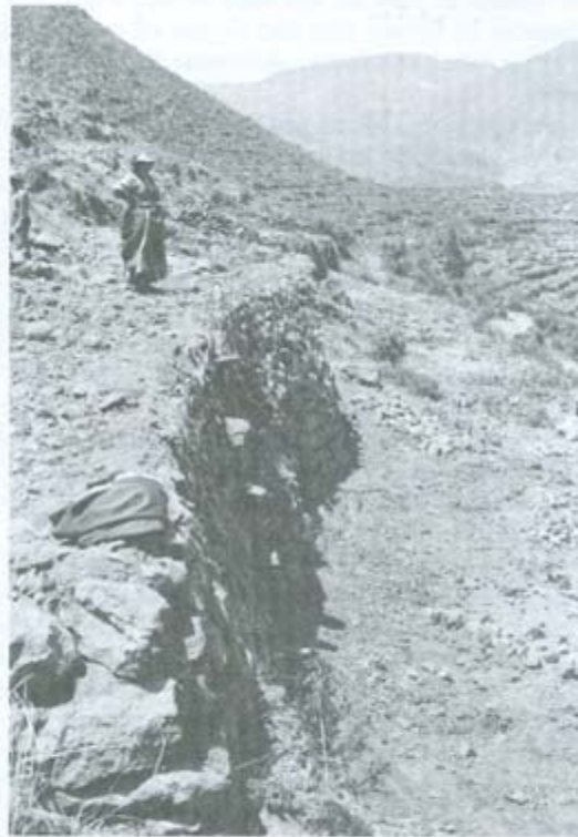
Fig. 8. Finished terrace with takilpus in foreground. Note inward inclination of wall for strength.
