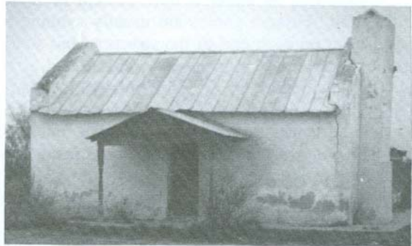
Fig. 5. House at Las Tiendas Ranch, northwest of Laredo in Webb County, Texas. Note the exterior chimney centered in one gable. Photo 1981, Texas Historical Commission WEB RUR 81/26/1, used with permission.
