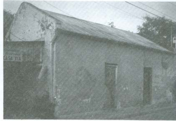
Fig. 7. Cafe, Grant Street in Laredo, Texas. Note the brick construction. Photo 1981, Texas Historical Commission WEB DO 81/10/34, used with permission.
