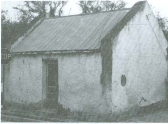
Fig. 2. One-room, square plan house, Grant Street, Laredo, Texas. Note the metal roof over shingles, the lack of windows, and plastering. Photo 1981, Texas Historical Commission, WEB DO 81/22/5, used with permission.
