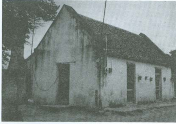
Fig. 6. Tranquiliño-Treviño house, 5th Street, Los Saenz, Starr County, Texas. Note the rectangular plan, multiple entrances, Spanish door on gable, and chimney attached to shed room. Photo 1981, Texas Historical Commission STA RUR 81/4/17A, used with permission.
