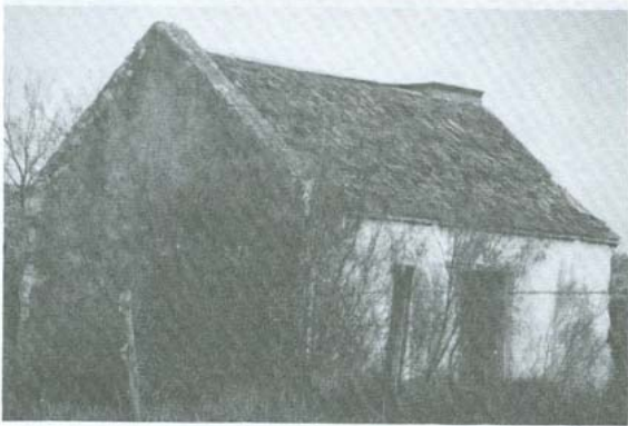
Fig. 4. House at Mirasoles Ranch, Starr County, Texas. Note the single parapet gable and the lack of windows. Photo 1981, Texas Historical Commission STA RUR 81/3/2A, used with permission.
